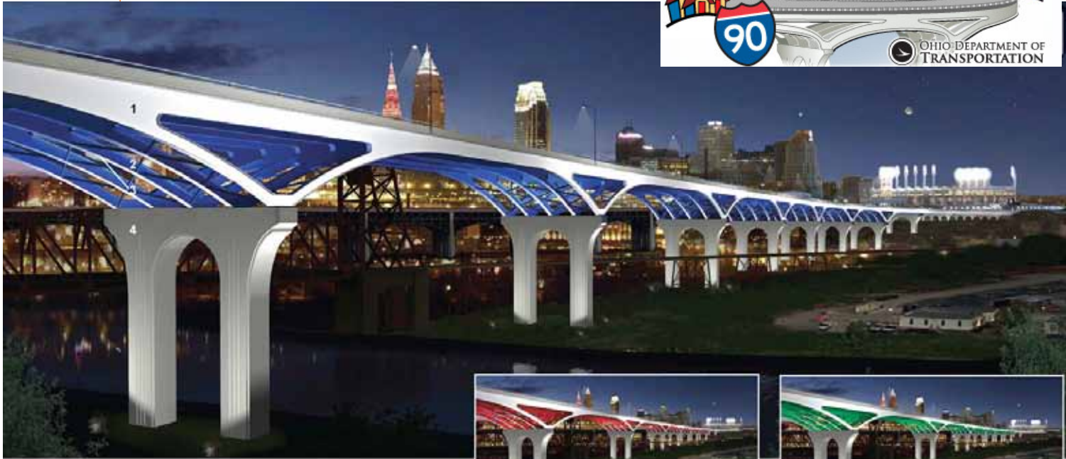
Night views of the new Innerbelt Bridge
